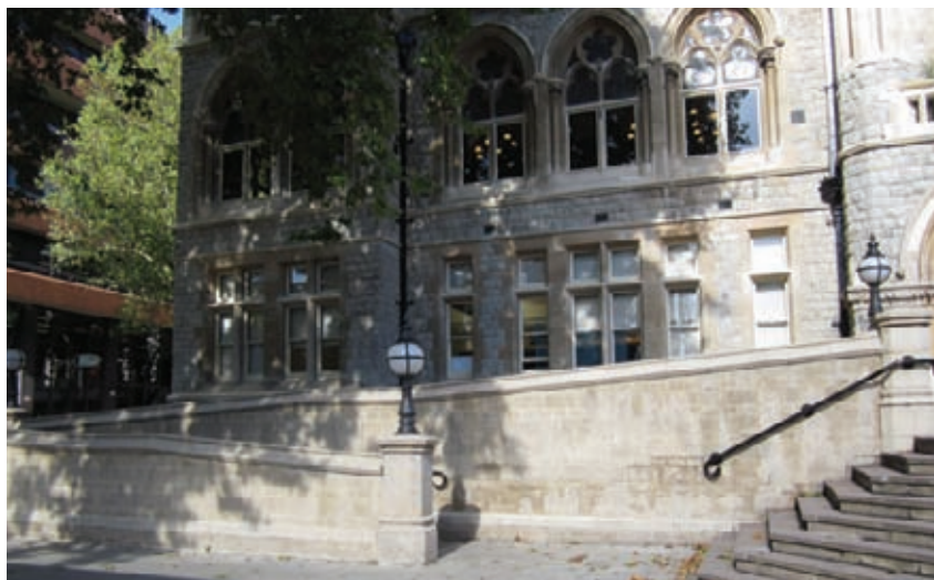
Asymmetrical elevations can accommodate alteration more easily. The addition of this significant ramp at Ealing Town Hall does not upset the balance of the overall composition and the design and use of materials is sympathetic.
