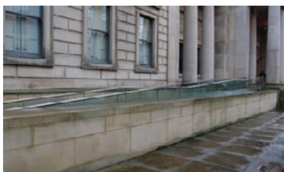
At Manchester Art Gallery the symmetrical composition of the main façade is not disturbed by the ramp, which rises to the portico entrance on one side only.
