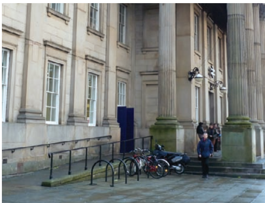
At Huddersfield station the asymmetry of a single ramp rising to the portico is insignificant when seen against the heroic scale of the larger design.
