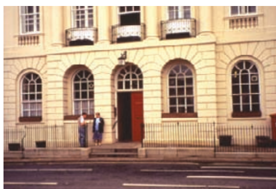
At Ripon Town Hall the whole pavement has been ramped up to threshold level over the original steps, part of a scheme that included the addition of a lift and accessible toilets inside. Railings have been added because of the increase in kerb height, but no handrail has been provided for the steps.
