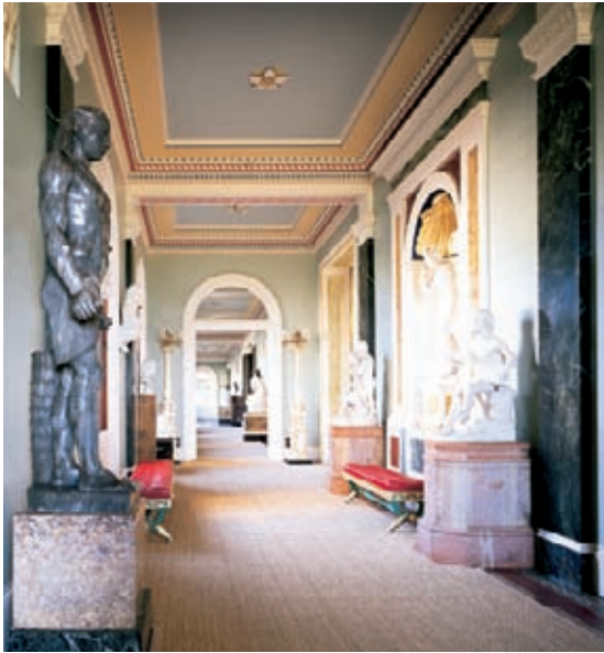
A Minton tile floor, such as this one underneath matting at Osborne House, is particularly vulnerable to both foot traffic and wheelchairs and needs to be protected.
