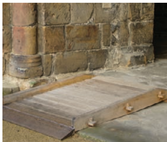
Removable timber ramps, such as this one at Richmond Castle in North Yorkshire, can provide access where a permanent intervention is not possible.
